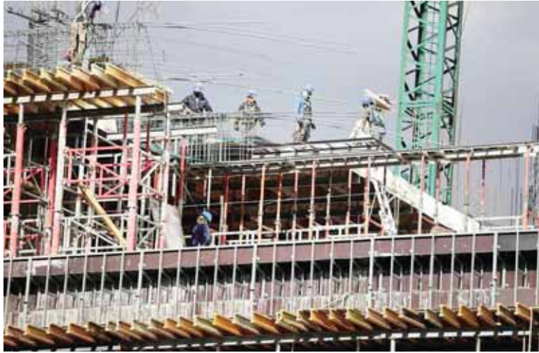
Workers are seen in a building construction in Mexico City. — Reuters
