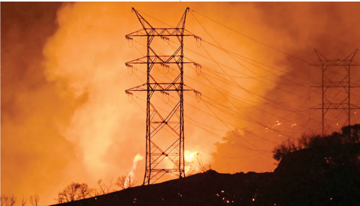
Flames and smoke are seen near power lines as the Palisades fire grows near the Mandeville Canyon neighborhood and Encino, California. — AFP
