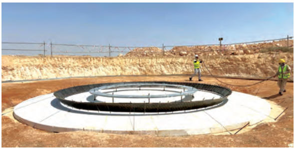
The base of a wind turbine being prepared at one of the wind farms under construction within PDO’s Block 6 licence.
