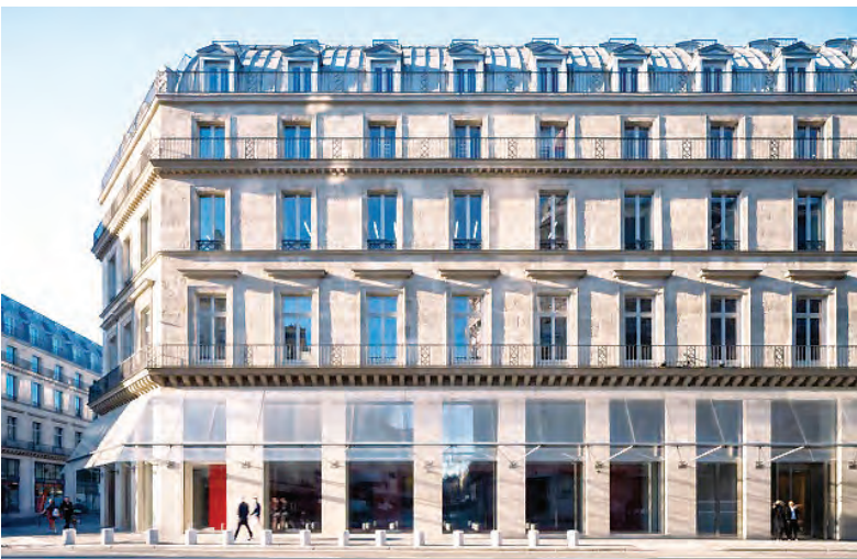
The new space is located at the Place du Palais-Royal, opposite the Louvre. — Foundation Cartier courtesy
