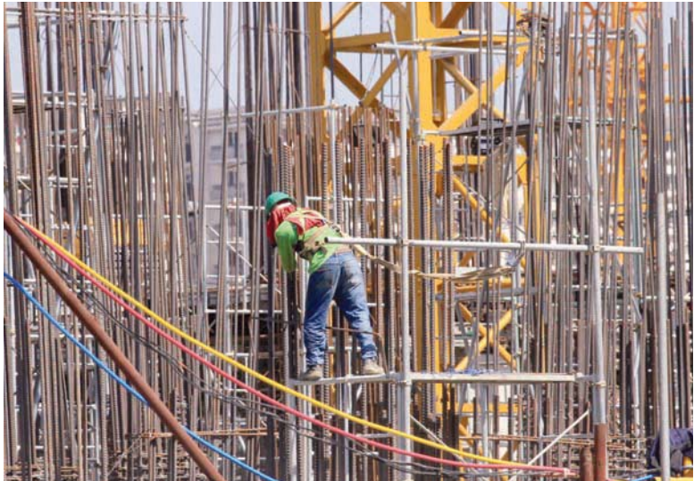
A worker installs steel rods at a construction site in Manila. – Reuters
