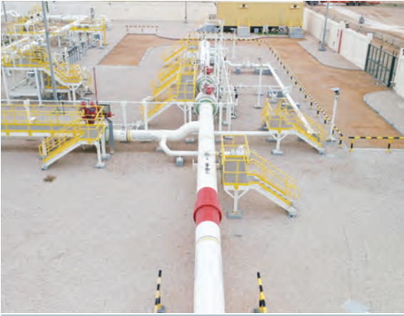
The new facility will help unlock new value from Oman's natural gas resources. Picture for illustration only.
