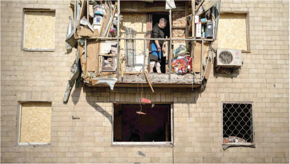
A man stands on a damaged balcony on Ukraine’s northeastern city of Kharkiv. — AFP
