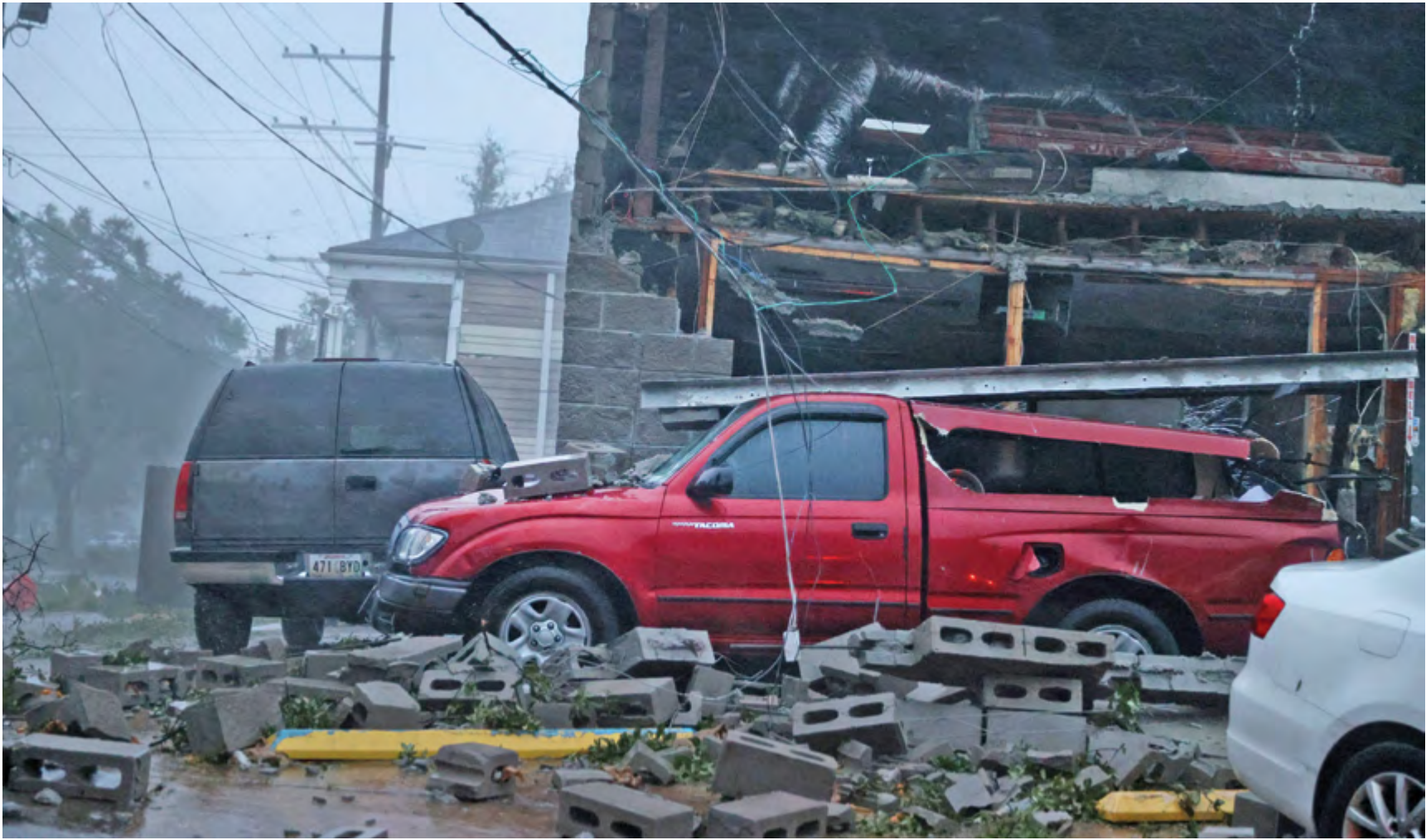
Damaged vehicles in front of a building collapsed during Hurricane Ida speak volumes about the devastation in New Orleans, Louisiana, on Sunday (AFP)
