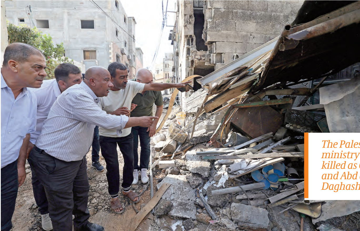
Residents inspect the damage at the Nur Shams refugee camp in the northern city of Tulkarem in the occupied West Bank on Sunday (AFP)
