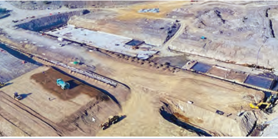
The project has progressed steadily since construction began in April 2025.
