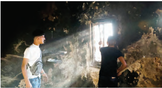
Palestinian men inspect a burnt-out room following an attack by Israeli settlers in Sarra near Nablus, the West Bank. — Reuters
