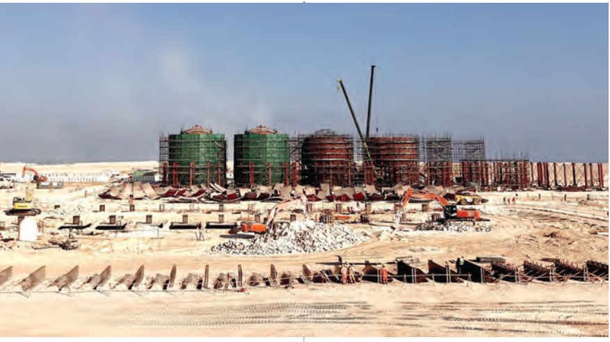
Tank capacity taking shape at Duqm SEZ as part of ACME Group's green ammonia project.
