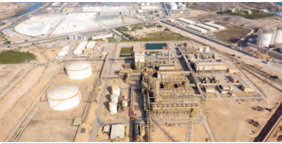
OQBI's integrated complex at Salalah produces methanol, ammonia and LPG
