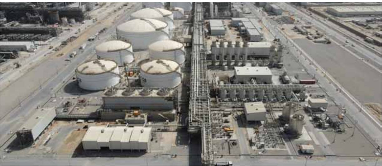
An overview of Duqm Refinery project. Image for illustration only.
