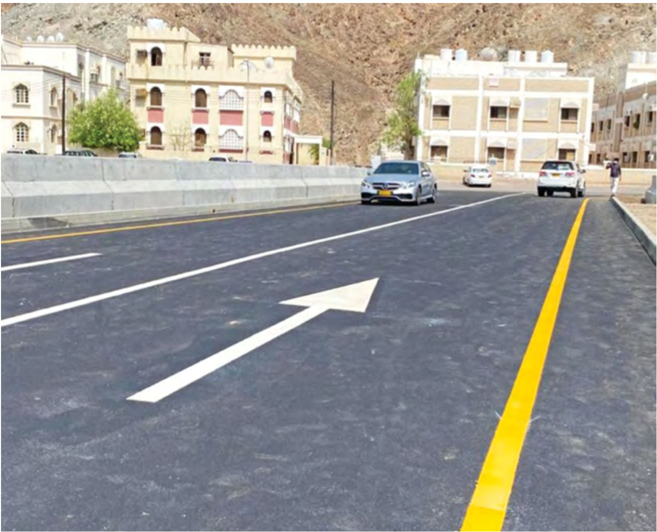
A long-awaited demand of Darsait residents has been met with the opening of a bridge over the wadi that often left people in the area cut off during rains. Muscat Municipality announced the opening of the bridge on Sunday. 'The project to construct a bridge with culverts over the wadi has been completed,' it stated. Following rains, the overflowing wadi inconvenienced residents and visitors to the area (Supplied photo)
