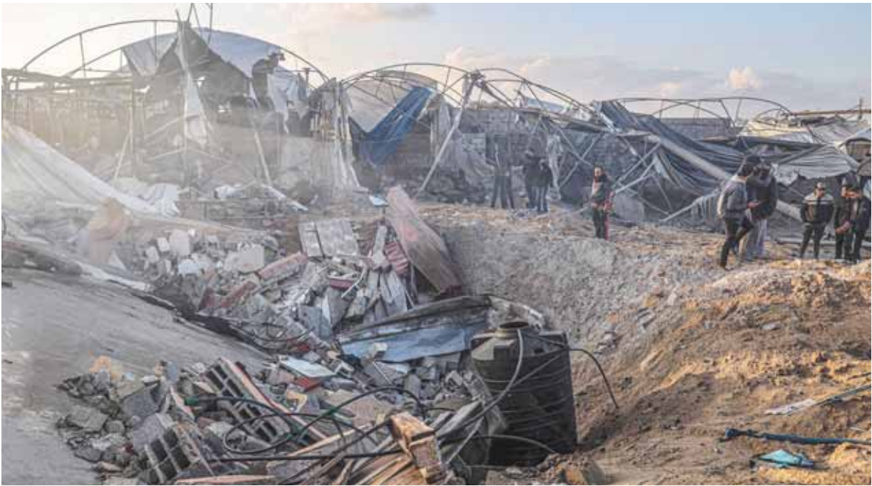
Palestinians inspect debris and rubble of a destroyed building following Israeli bombardments in Rafah. – AFP
