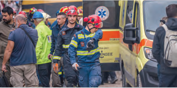
Emergency personnel work after an old building partially collapsed in the Plaka area of central Athens. — AFP
