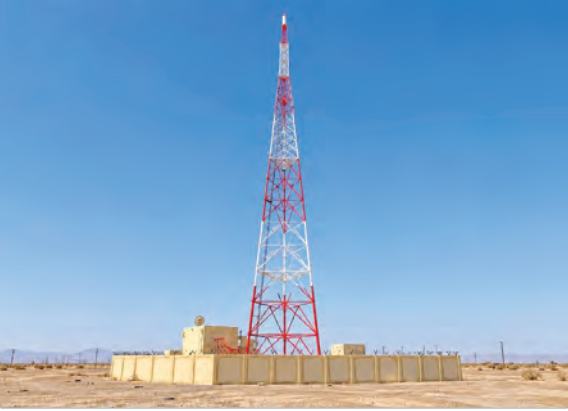
The first phase of the project involved the execution of 69 television transmission stations distributed across various governorates and wilayats of the Sultanate of Oman.
