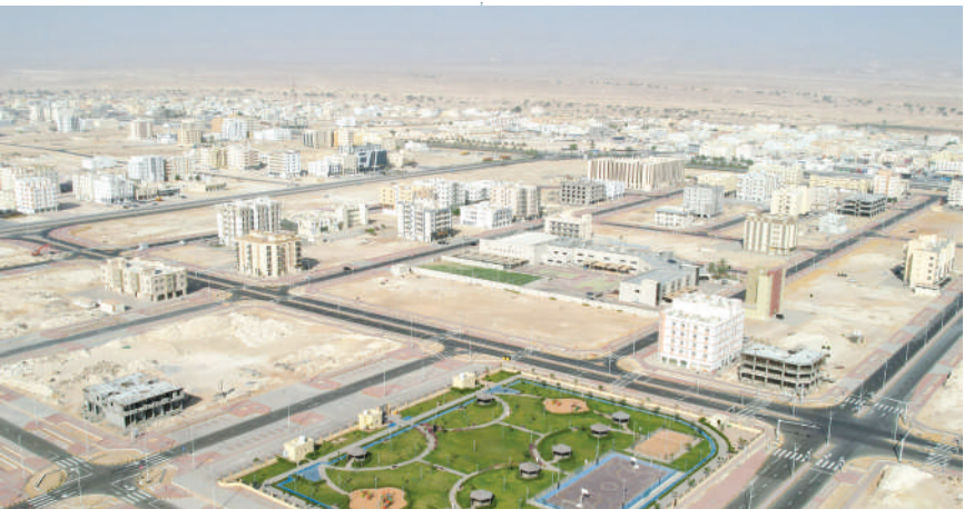
Tatweer manages a wide range of public assets and facilities across Duqm.
