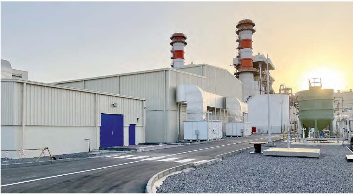
Barka V desalination plant nearing completion in Al Batinah South Governorate.
