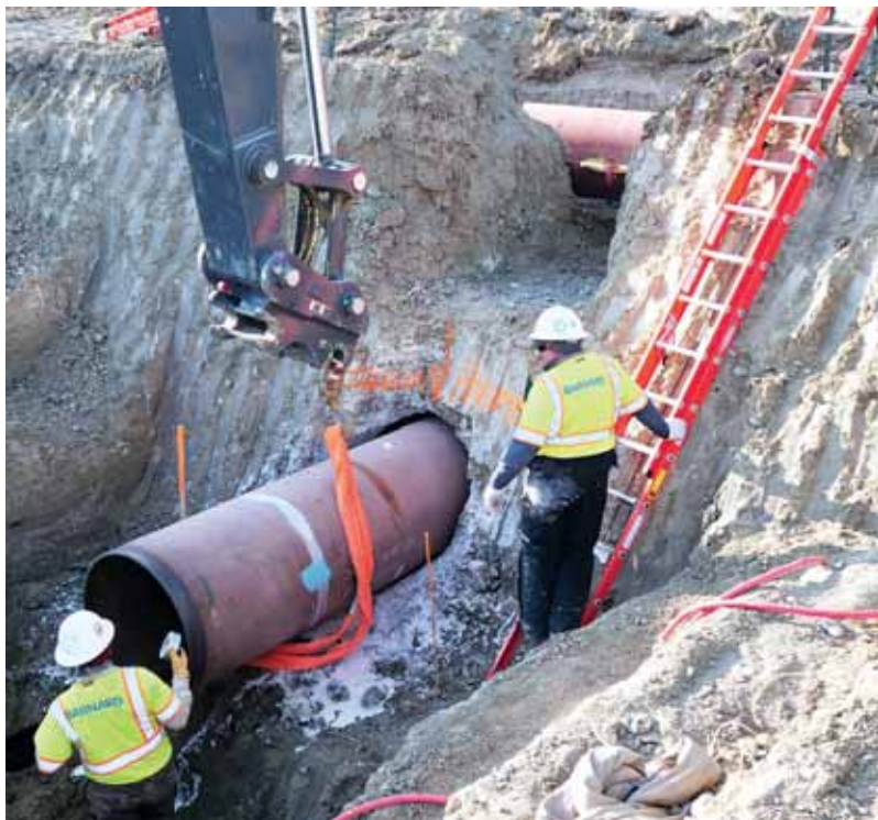
Men work on the construction on the Keystone XL pipeline in Montana. — AFP
