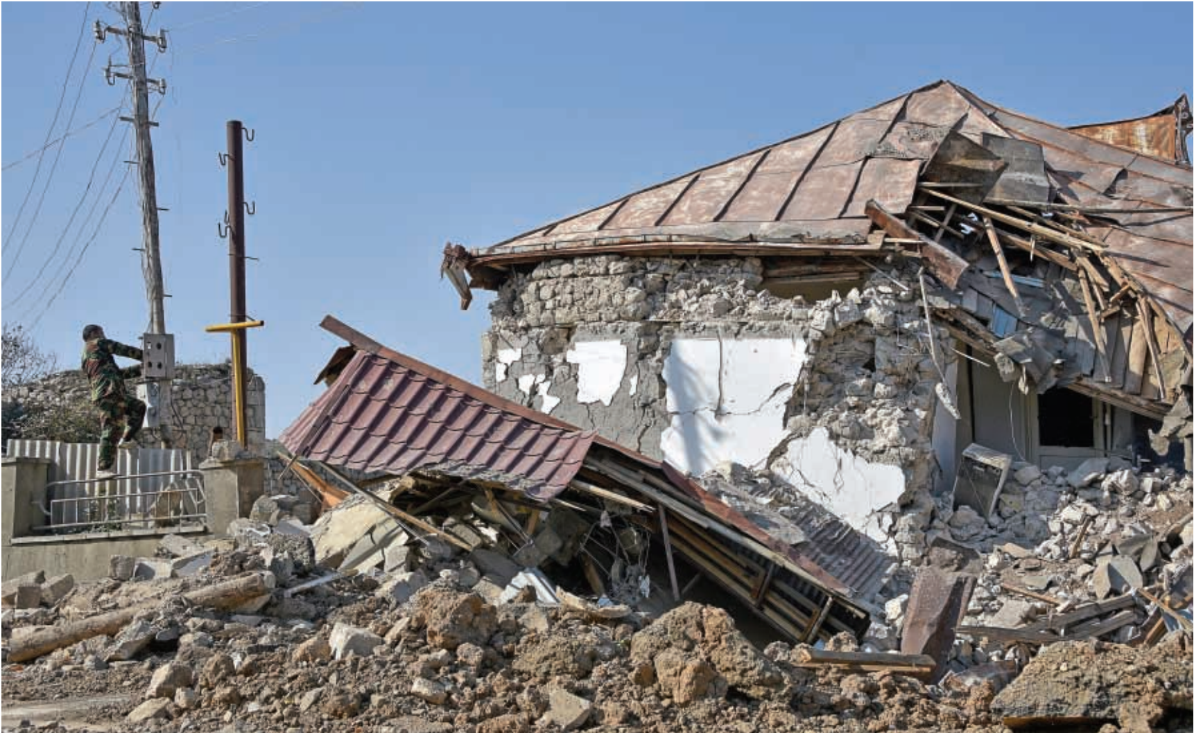
This file photo shows a man fixing electricity cables next to a destroyed house in the city of Shusha, some 15km from Nagorno-Karabakh province's capital Stepanakert, on November 1 (AFP)
