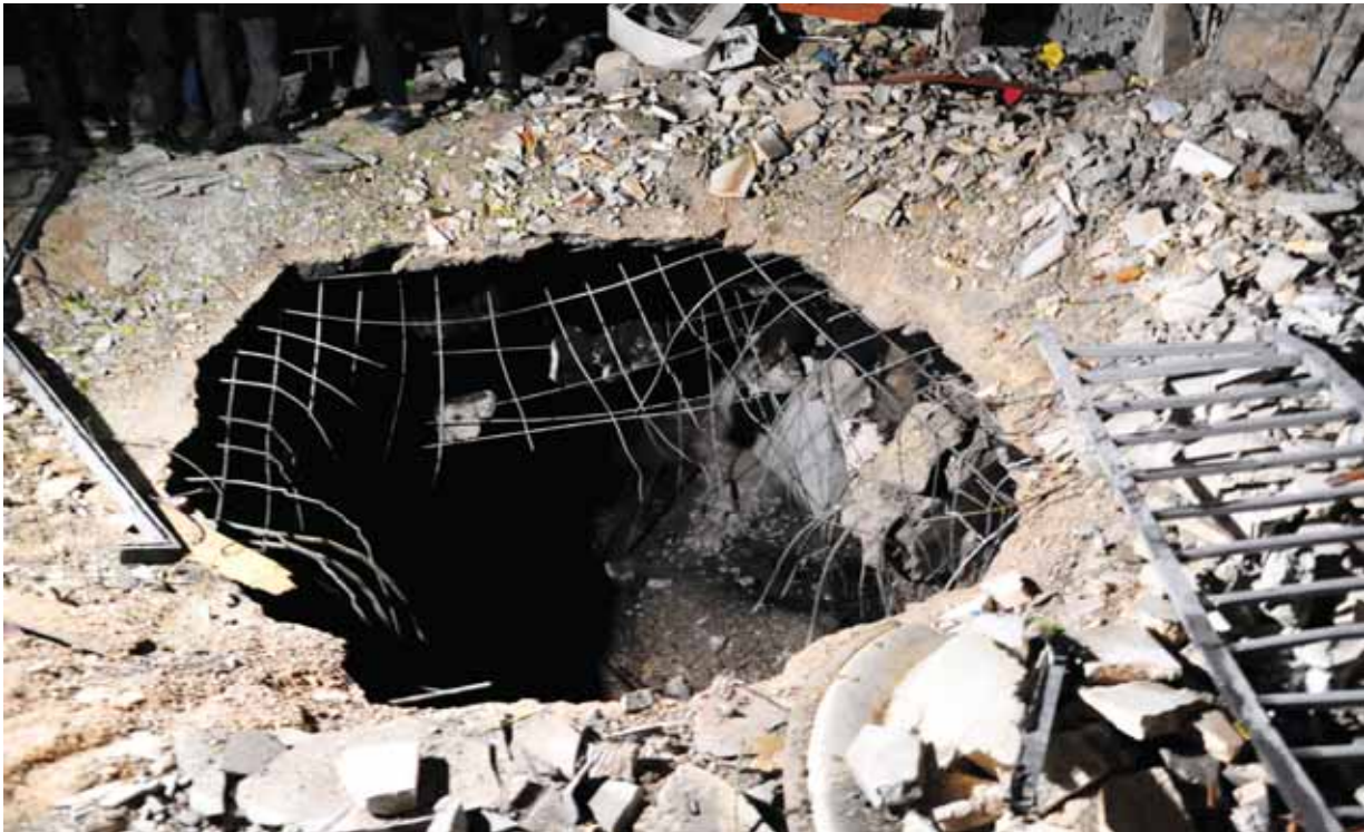
A view shows damage at the site of a rocket attack, in central Damascus's Kafr Sousa neighbourhood of Syria. — Reuters
