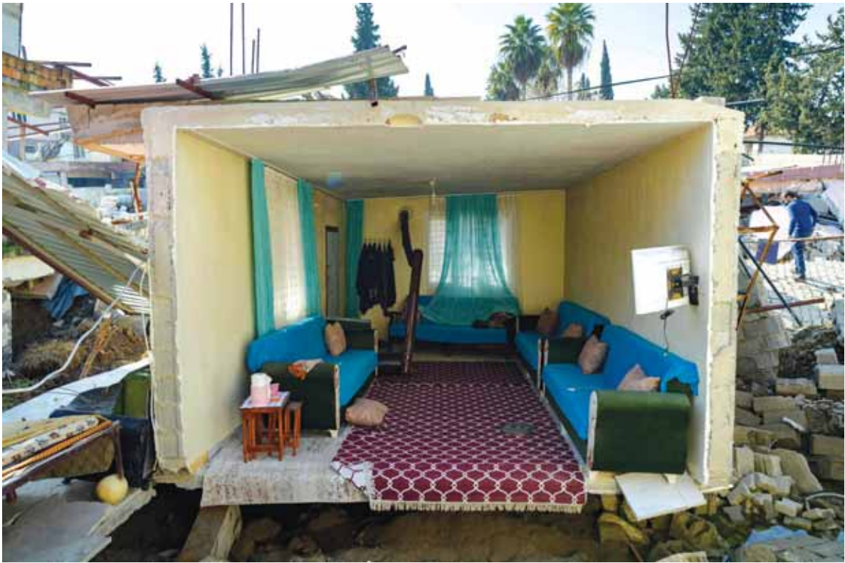
A view of a living room in Demirkopru, a small destroyed Turkish village now divided by a large crack in Hatay. — AFP
