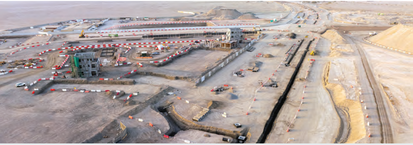
Ongoing construction at one of the project sites in Sultan Haitham City.
