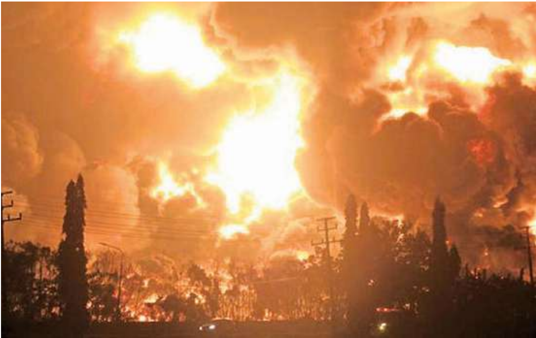
MASSIVE FIRE: A column of black smoke rose from the state-run Pertamina Balongan Refinery in West Java, about 225 km (140 miles) east of Jakarta
