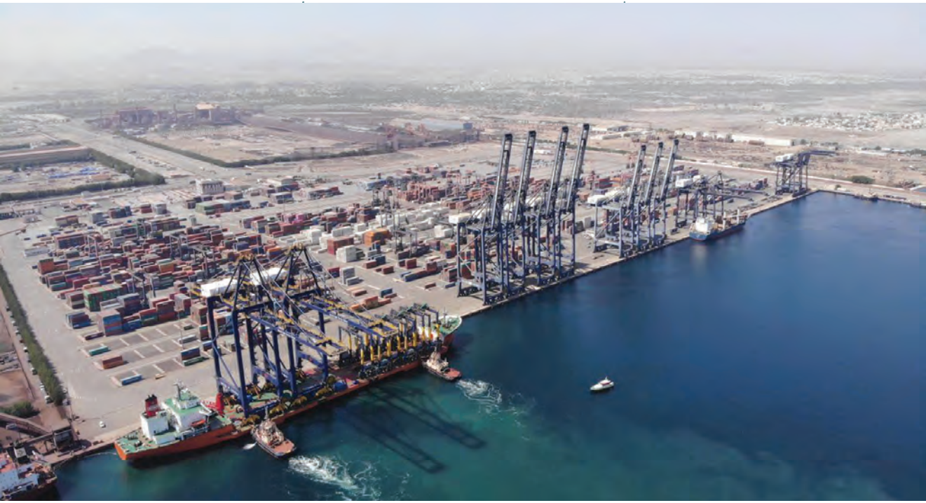
SOHAR Port and Freezone is described as Oman’s main commercial and industrial gateway.
