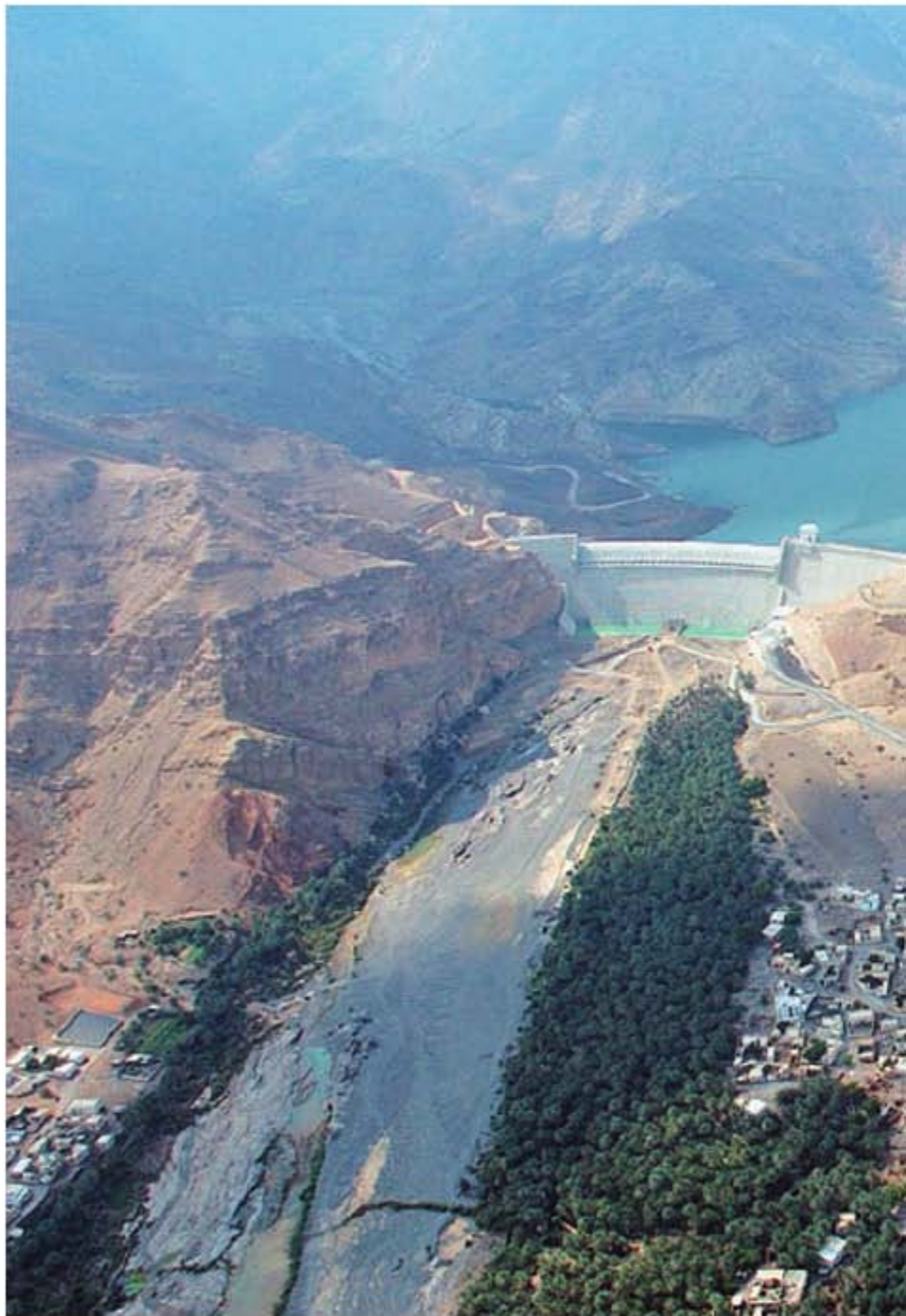
Aerial view of Wadi Dayqah Dam. This project involved the construction of two dams located just upstream of Mazara village, ie the Main Dam across the Wadi Dayqah, and a Saddle Dam on the depression in the left rim of the reservoir.
