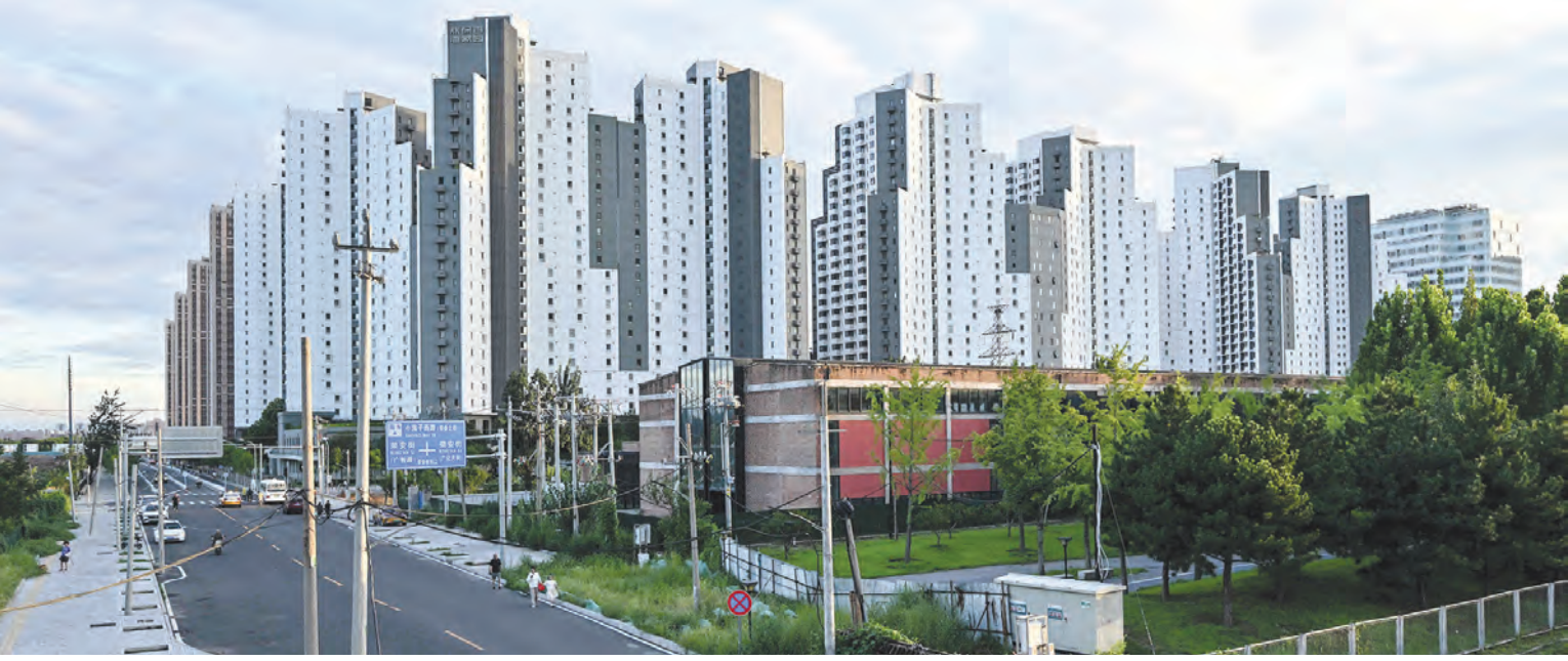
A general view shows the Baiziwan Social Housing project, a subsidised residential compound for low-income communities. — AFP
