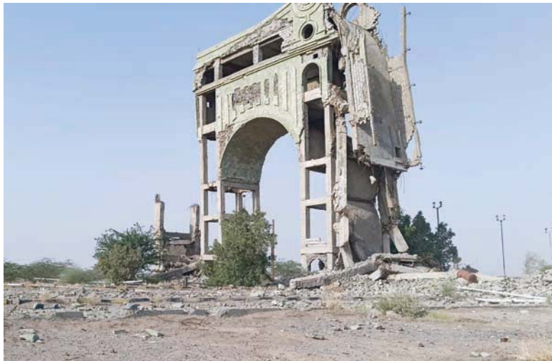
A view of an arch damaged by clashes is seen on the outskirts of the Red Sea port city of Hodeidah. – Reuters
