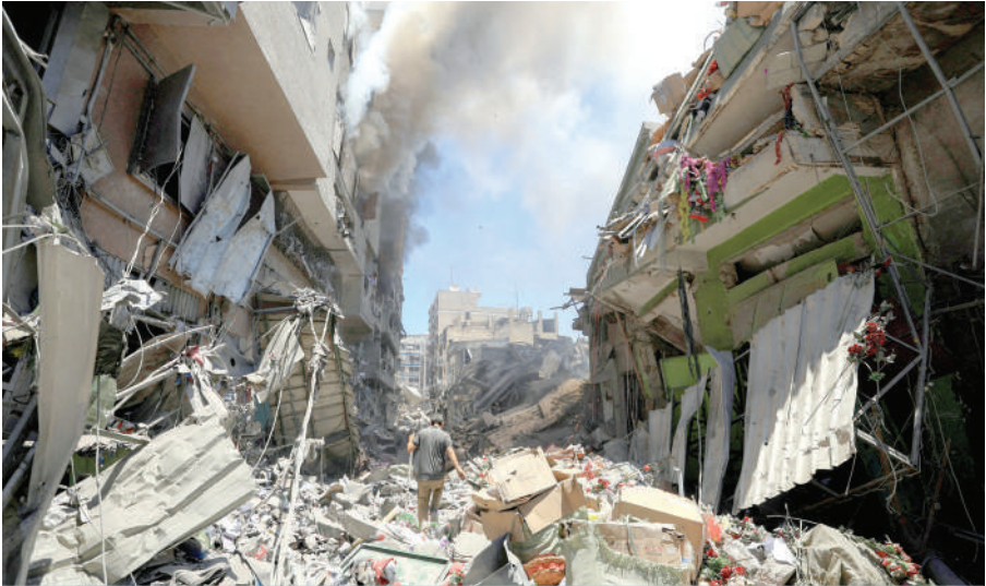
Smoke rises as a Palestinian man inspects the site of Israeli strikes on buildings at Gaza’s Old City market on Wednesday. — Reuters
