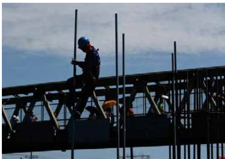
A worker assembles a pole at a construction site of the Metro Rail Transit (MRT) on Commonwealth Avenue in Quezon City, Philippines. — Reuters
