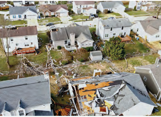
Debris lies around damaged houses after a tornado touched down in Florissant, Missouri, US. — Reuters
