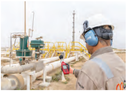
The 193-km pipeline will boost the capacity of OQGN's gas supply system
