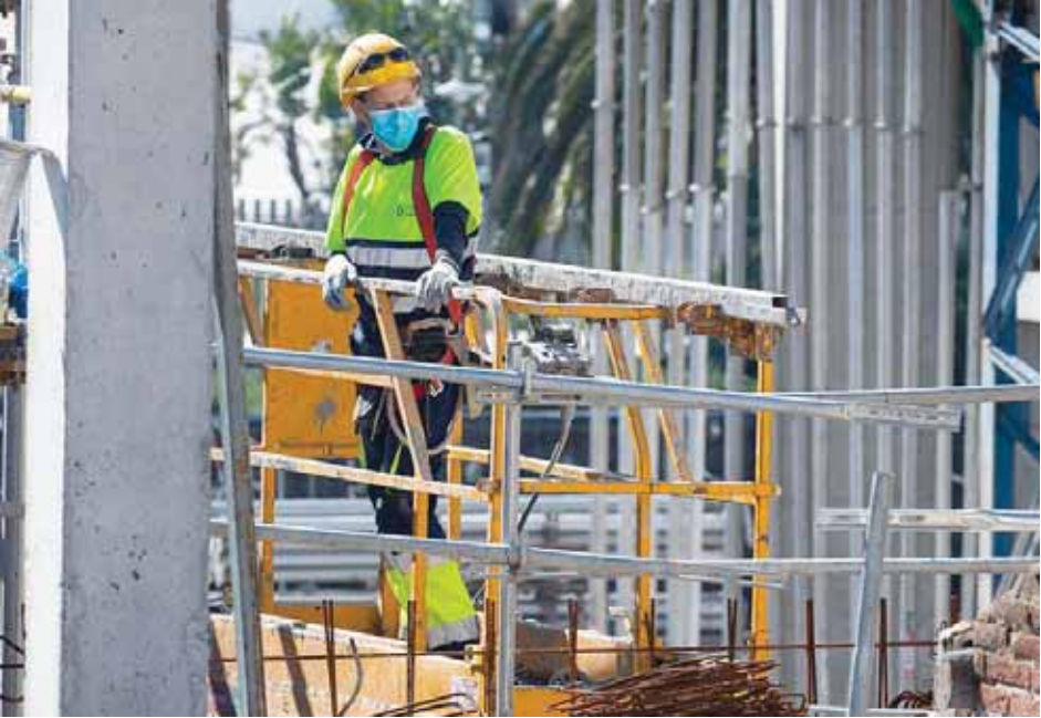
Construction workers return to work under Covid-19 conditions.
