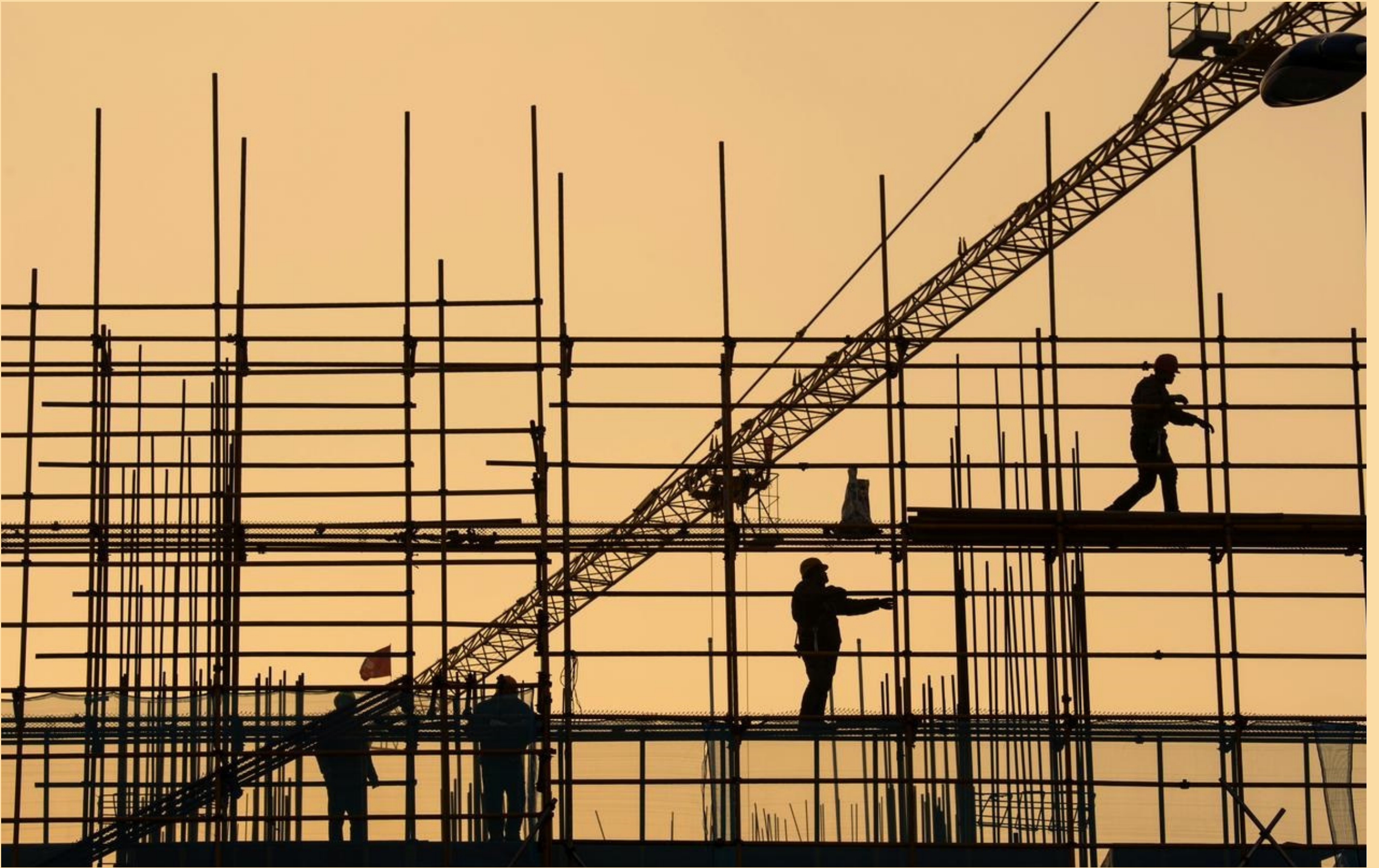
Workers are seen on scaffolding at a construction site in Nantong, Jiangsu province, China. — Reuters
