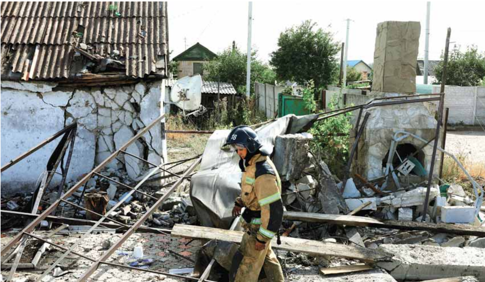
A firefighter works in the yard of a destroyed house following the shelling, in the Donetsk region.
