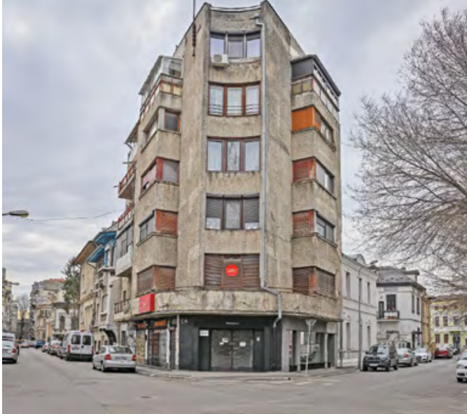
An interbellic block of flats with a red sign indicating that the building has been classified as seismic risk class I is seen in Bucharest on March 18 (AFP)
