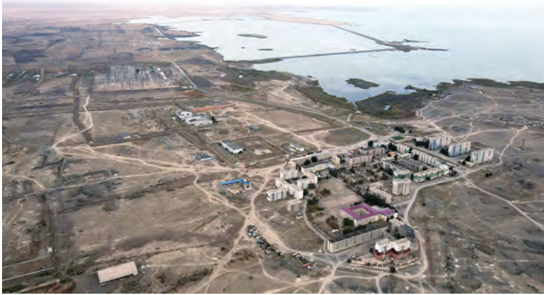
An aerial view shows the village of Ulken and the proposed nuclear power plant site near the village of Ulken. — AFP
