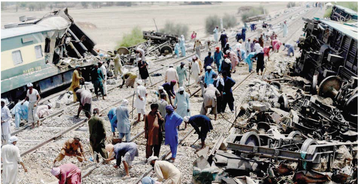
Workers repair a railway track near the wreckage of a train in Daharki on Wednesday, two days after a inter-city train ploughed into another express that had derailed killing at least 63 people. — AFP
