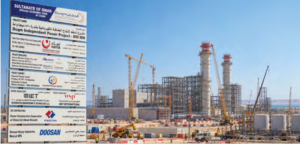
Visualisation of Coastal Power's 890 MW CCGT power plant under construction at Al Duqm.
