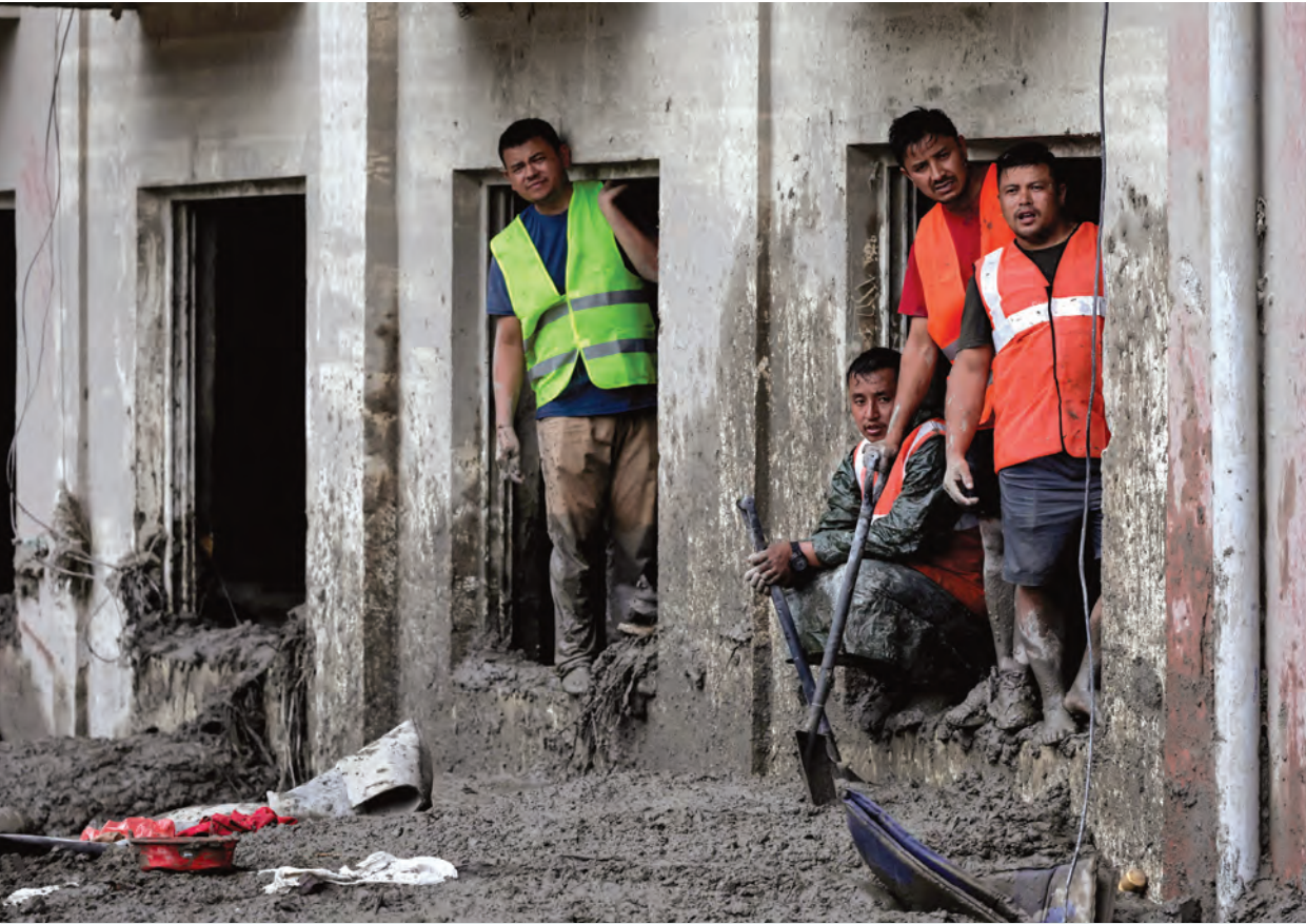
Rescue personnel look through the window of a damaged building in Devighat, Nuwakot, Nepal. — Reuters
