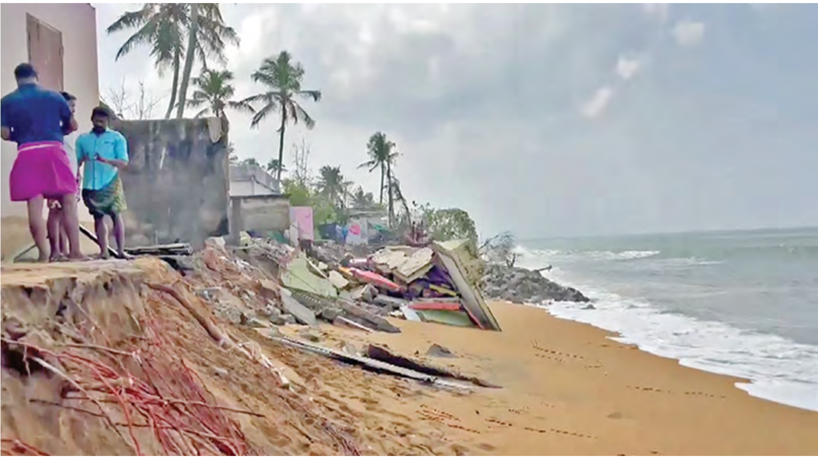
People stand near the houses damaged by the advancing sea and violent waves in the coastal city of Kollam in the southern state of Kerala on Tuesday (ANI)
