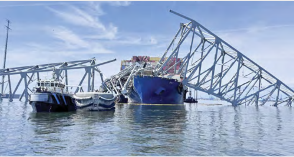
A file picture of the fallen Francis Scott Key Bridge in Baltimore, US
