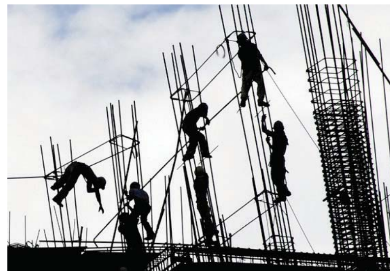
Construction workers are seen at Bonifacio global city in Philippines. — Reuters
