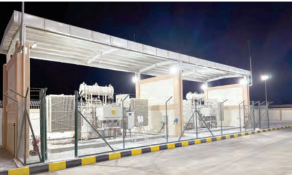
The projects include new and upgraded substations, additional 33-kV feeders and network automation.
