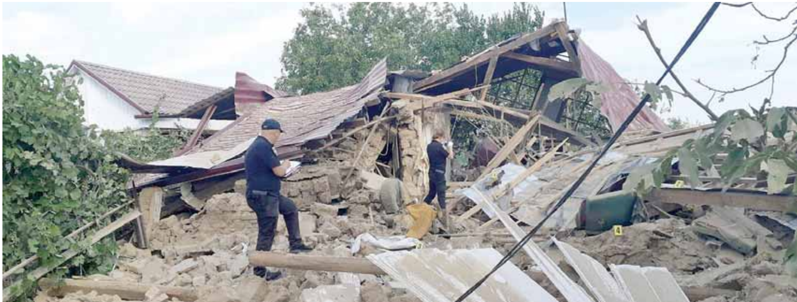
Police officers inspect a residential house destroyed by a Russian military strike in the location given as Marhanets town, in Dnipropetrovsk region, on Wednesday. — Reuters
