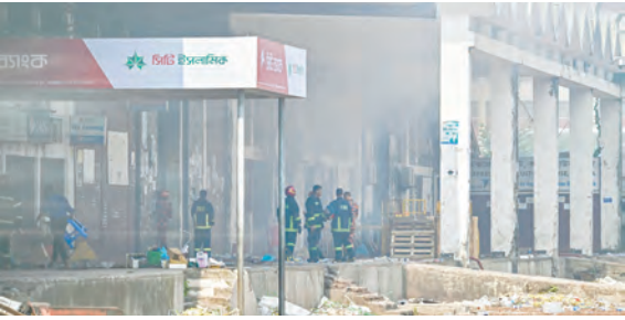
Firefighters inspect the damaged terminal of Hazrat Shahjalal International Airport in Dhaka. — AFP
