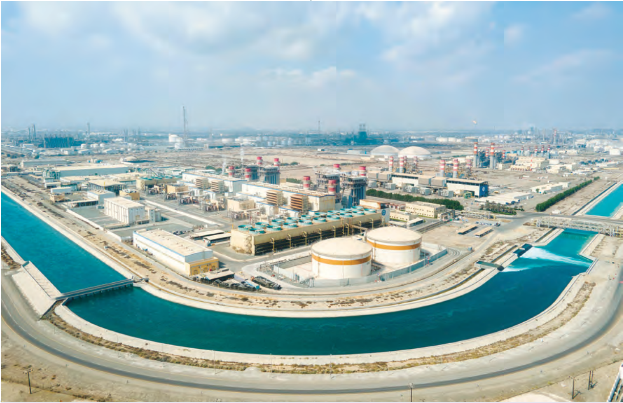
Construction is progressing on a major infrastructure expansion covering 670 hectares
