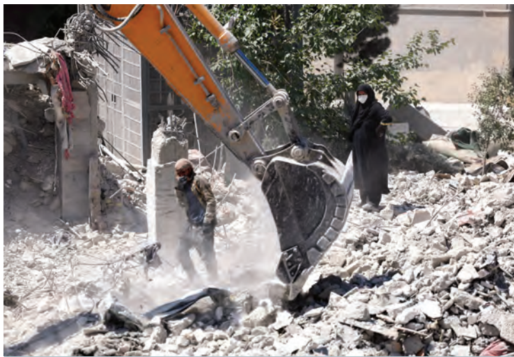
A woman stands among the rubble of her house, which was damaged in a strike, in Tehran, Iran. — Reuters
