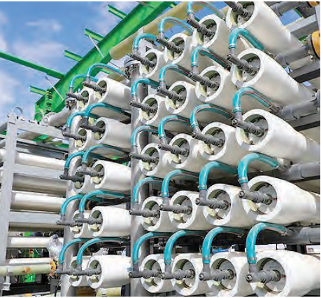
RO membranes are the core component of modern desalination plants.
