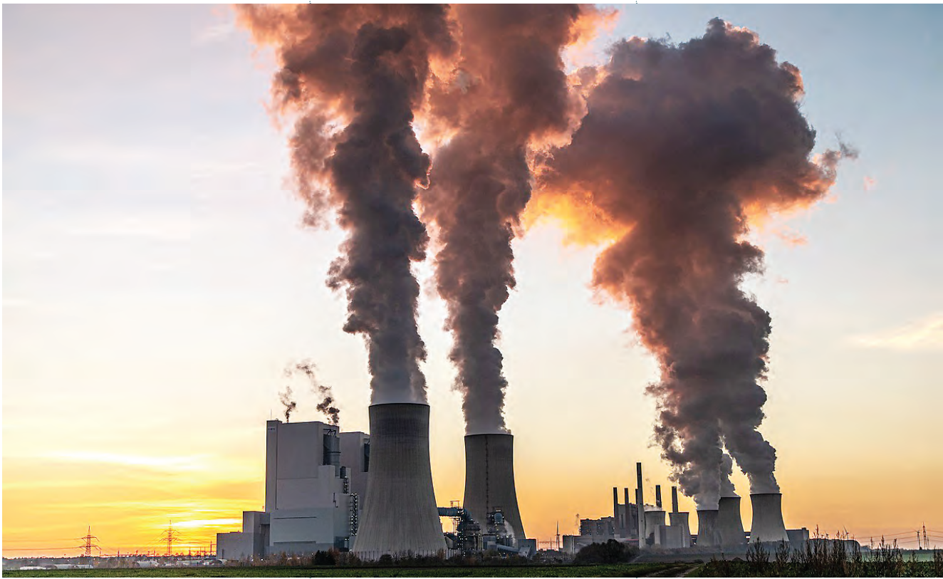
Northern Lights has an annual CO 2 storage capacity of 1.5 million tonnes. — AFP
