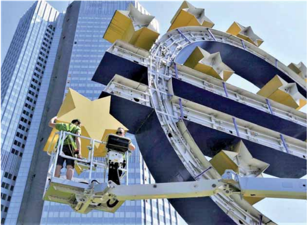
Workers dismantle the large Euro sign sculpture for maintenance, in front of the headquarters of ECB in Frankfurt. — Reuters
