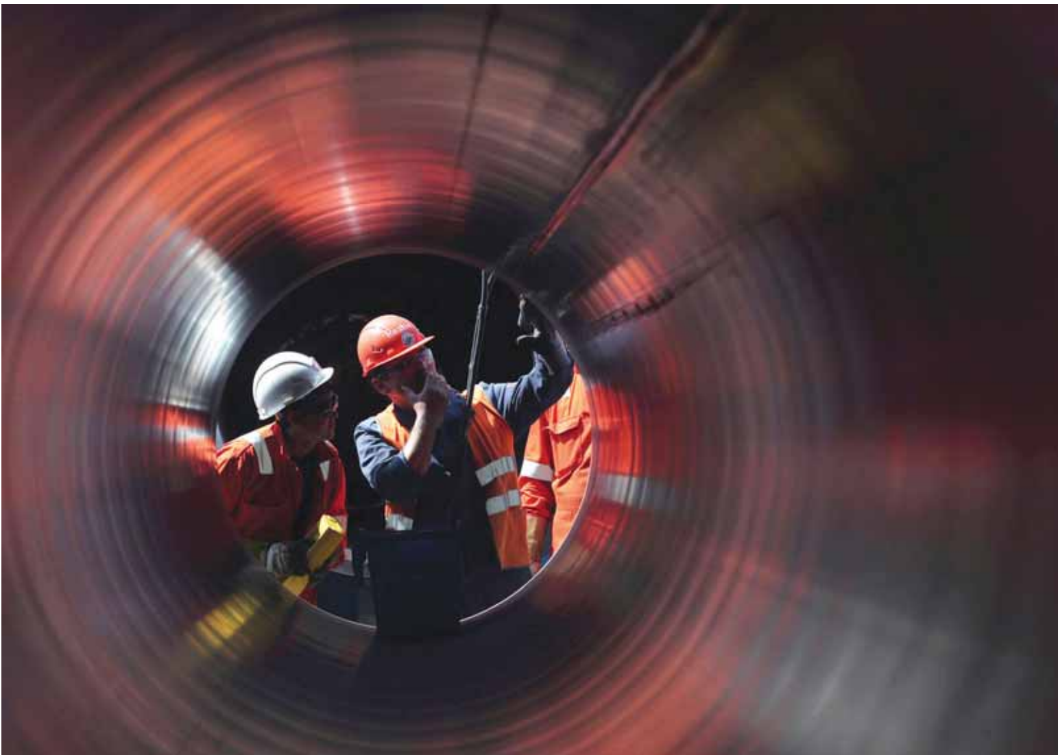
STREAMING WORKERS Workers are seen through a pipe at the construction site of the Nord Stream 2 gas pipeline, near the town of Kingisepp, Leningrad region, Russia. Beginning exports via the Nord Stream 2 pipeline under the Baltic Sea would lead to a reduction in gas prices in Europe, Russian President Vladimir Putin was quoted as saying by local news agencies on Friday. Nord Stream 2, completed in September, has faced resistance from the United States and several countries including Poland and Ukraine, which say it will increase Russia's leverage over Europe. — Reuters
