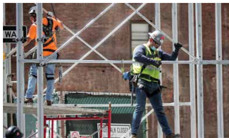
Construction workers assemble a scaffold at a job site in New York. — Reuters
