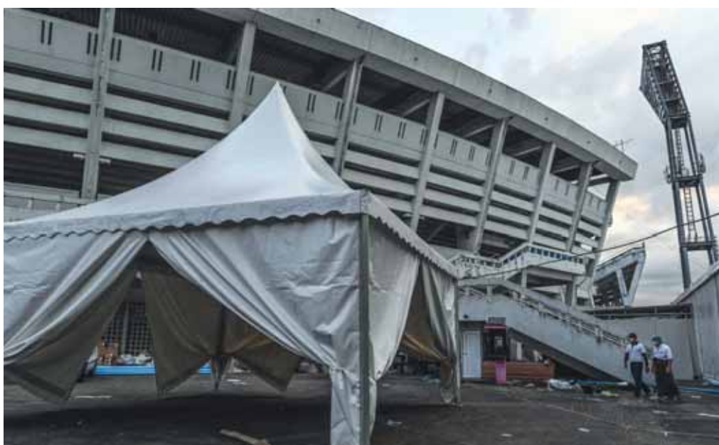
An under construction emergency building to be used as an Intensive Care Unit (ICU) for COVID-19 coronavirus patients at a football stadium in Yangon. — AFP
