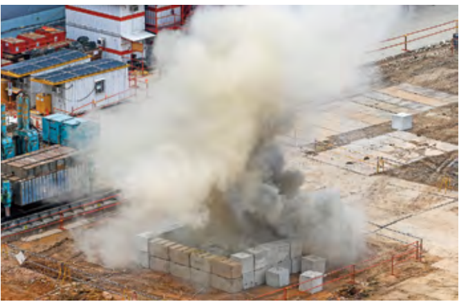
Smoke rises after a 100kg World War II-era aerial bomb is detonated at a construction site in Singapore on Tuesday (AFP)
