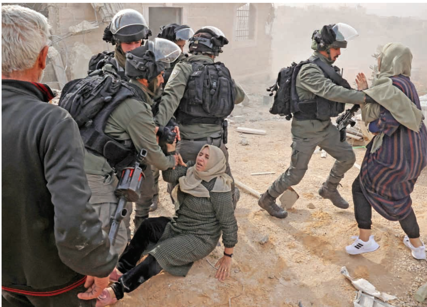
Palestinians are blocked by Israeli security forces as they try to stop the demolition of their home, located within the 'Area C' of the occupied West Bank, where Israel retains full control over planning and construction, in the town of Hebron on Tuesday (AFP)
