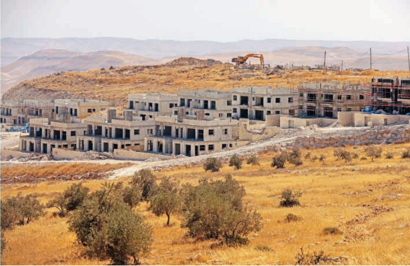
This file photo shows new houses under construction in the Nokdim settlement in the Israeli occupied West Bank, on October 13 last year (AFP)
